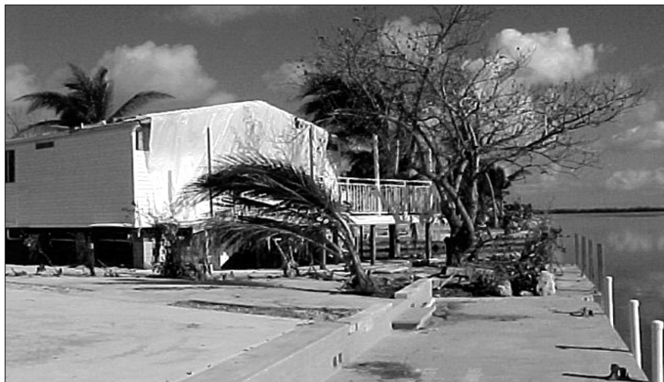
Figure 1-5. Manufactured home in Cudjoe Key, Florida, built and installed after 1994, survived Hurricane Georges with only minor damage caused by the loss of an awning. The older manufactured home on the lot next door was destroyed by high winds and coastal surge.
