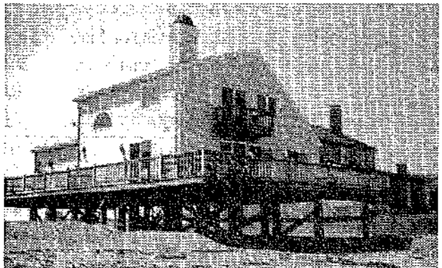
Flexible connections between building support beams and wooden piles allow adjustments to be made to account for imperfect pile driving.
