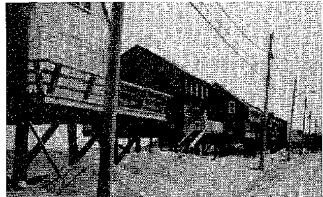
Many homes in Sandwich, Massachusetts, were relocated landward on their existing lots after severe dune erosion from an October 1991 Northeaster.
